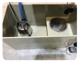
90 L. Buffer tank with filter basket and pump
